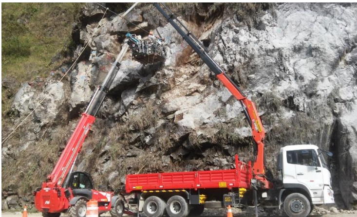
Photography 1. Slope pre-reinforcement.
