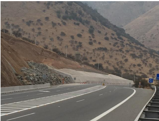
Figure 13. Final aspect of the motorway slope
