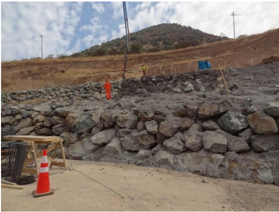
Figure 12. Detail of the grouting of the rockfill
