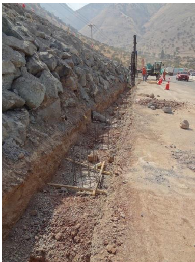
Figure 10. Execution of the toe retaining wall with reinforced piles
