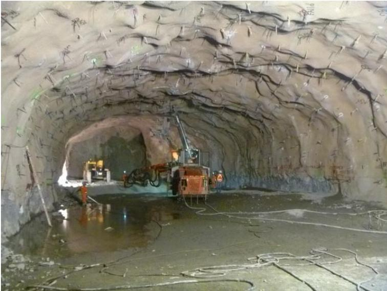
**Fig. 14** Powerhouse excavation. Bench I (Crown)
