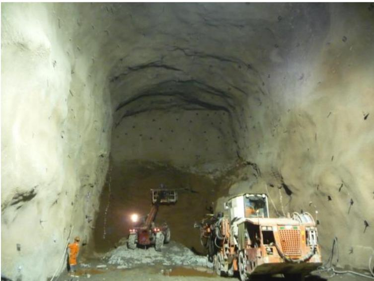
**Fig. 15** Transformer Cavern Excavation
