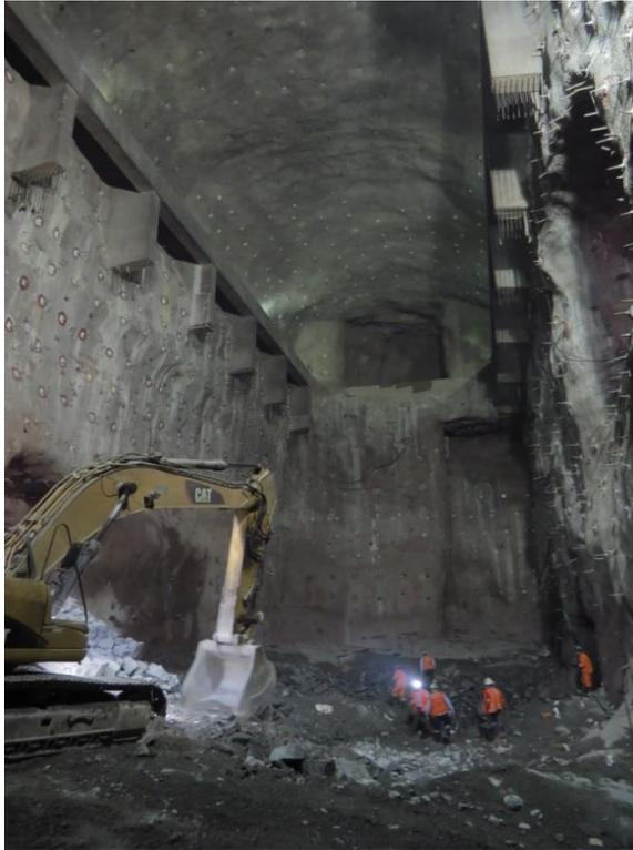
**Fig. 16** Powerhouse Excavation. Bench VI
