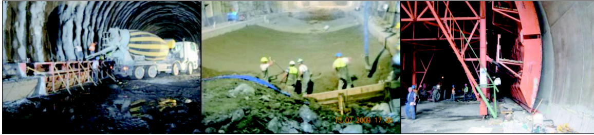
Figure 3. Overview of some phases in lining conventional tunnels
