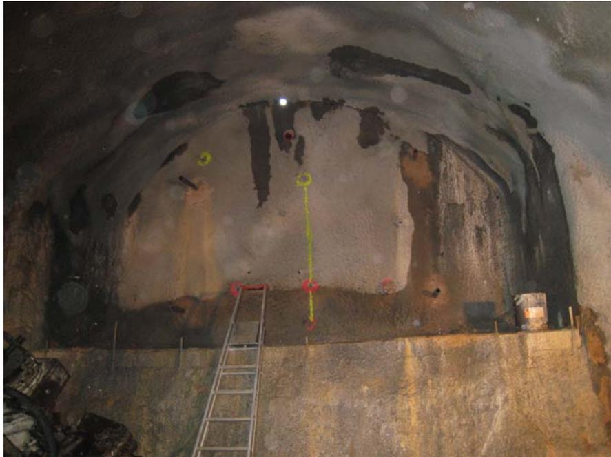
*Photo 6 – Drainage from the tunnel face with horizontal holes*
