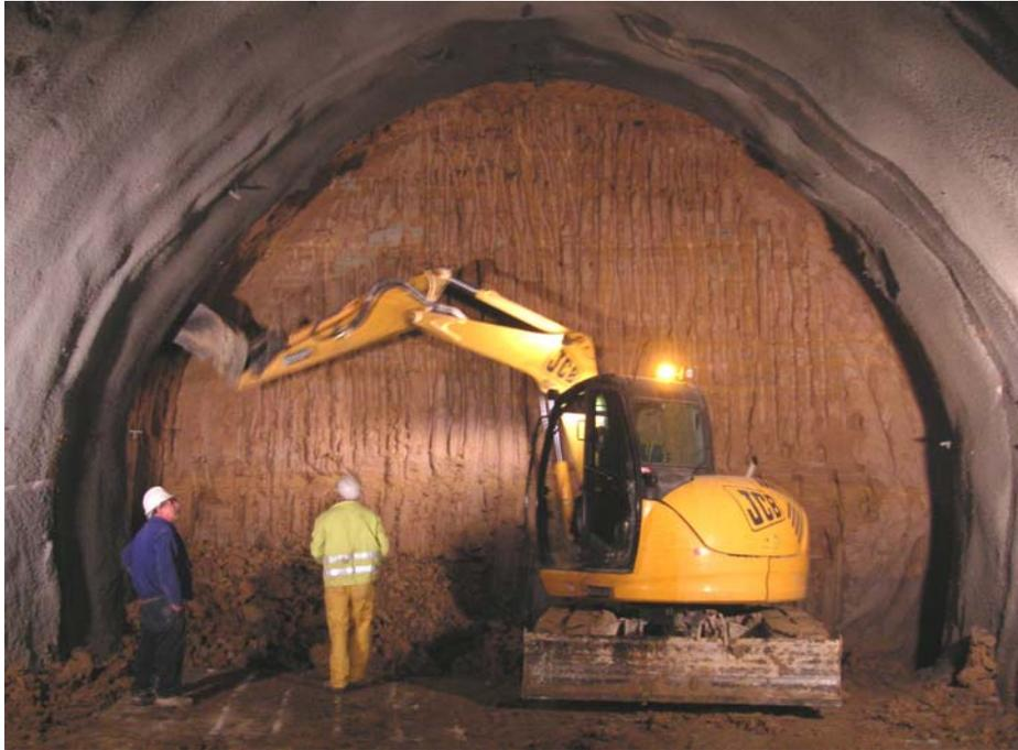
*Photo 2 - Claystones and silts, impermeable and stable face*
