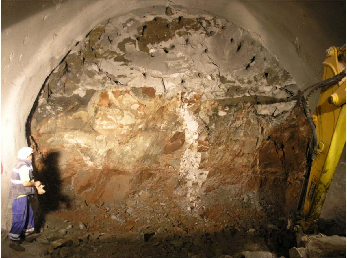
*Photo 8– Soil improved by jet-grouting over a rock layer*
