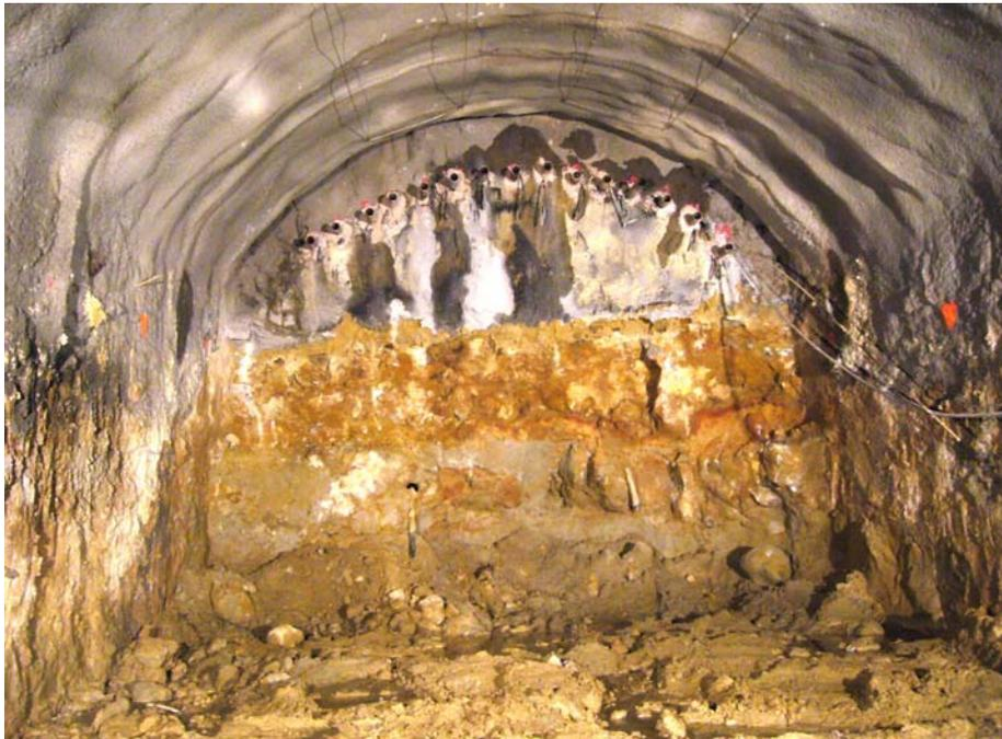
*Photo 3 - Heterogeneous permeable blocks and silts that produce an unstable face*
