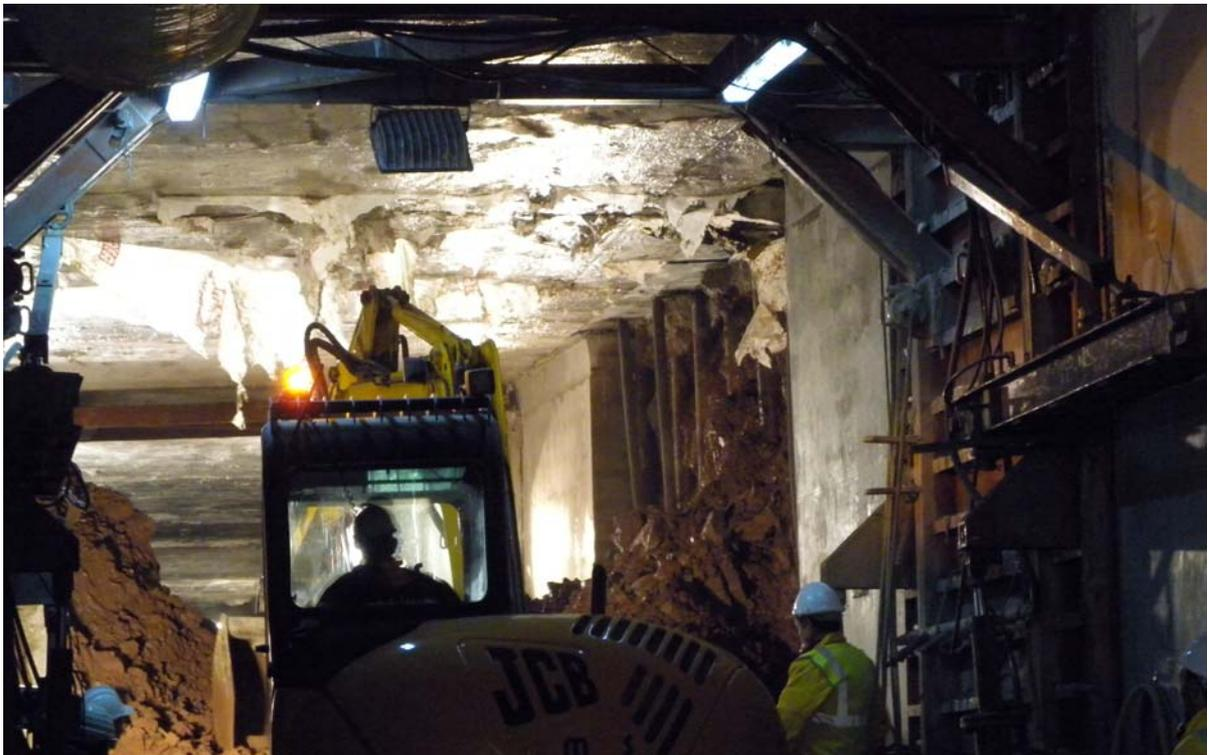
*Photo 9 – Detail of the breakthrough of the lower phase*
