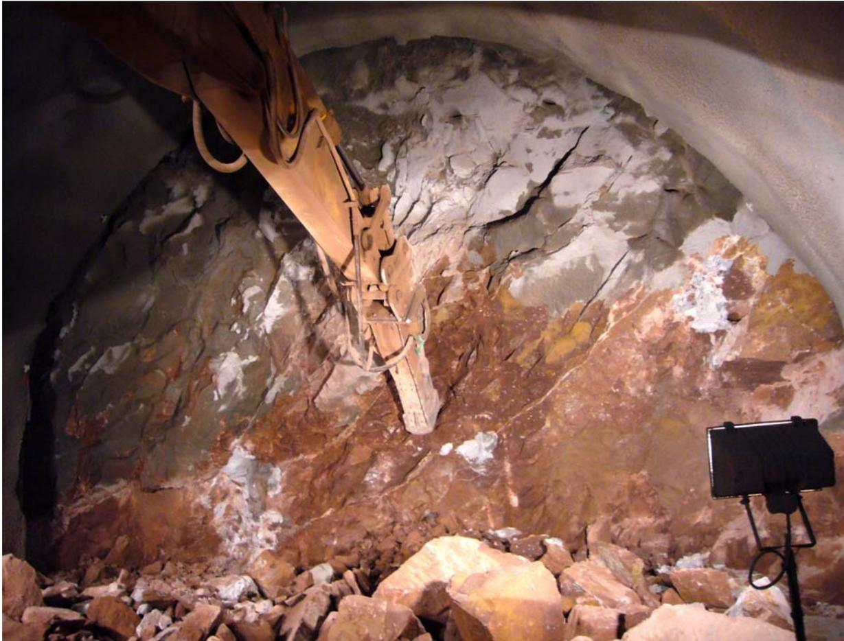
*Photo 4 - Strong and permeable sandstones that produce a stable face*
