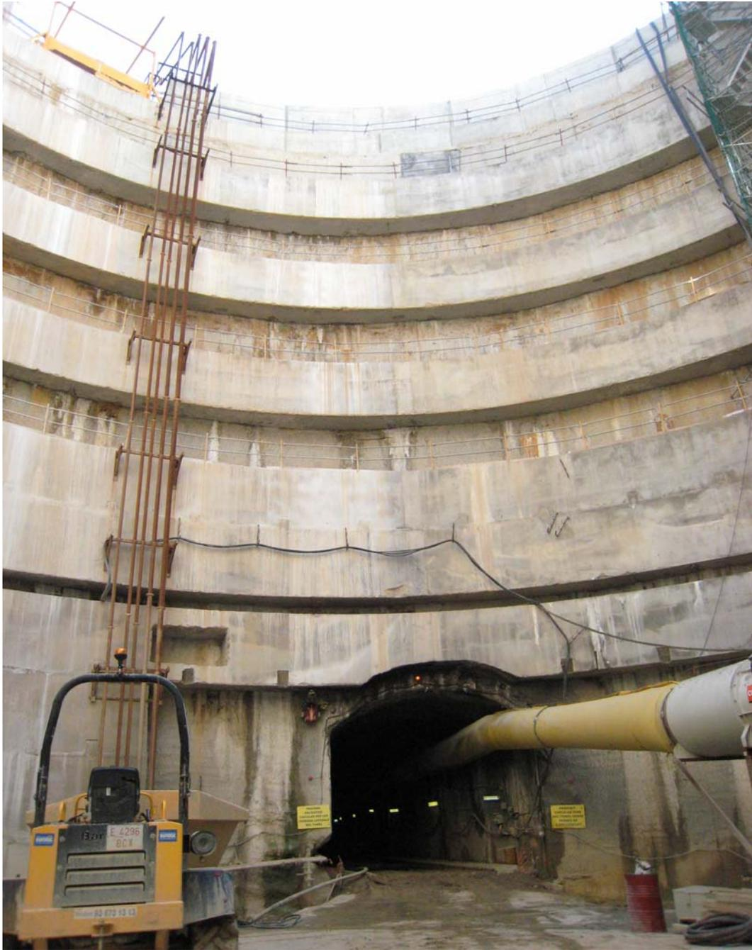
*Photo 5– Beginning of the tunnel construction from the Bifurcation Shaft*
