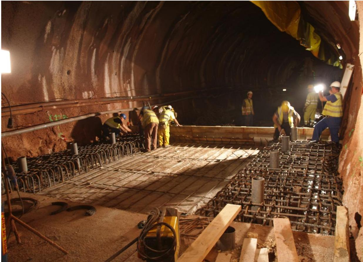
*Photo 7 – Construction of the intermediate concrete slab that permits to close the upper phase of the tunnel*
