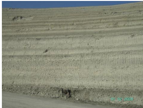
Figure 5. General aspect of the bedding in the marls and detail of one of those planes showing a millimetrical displacement.
