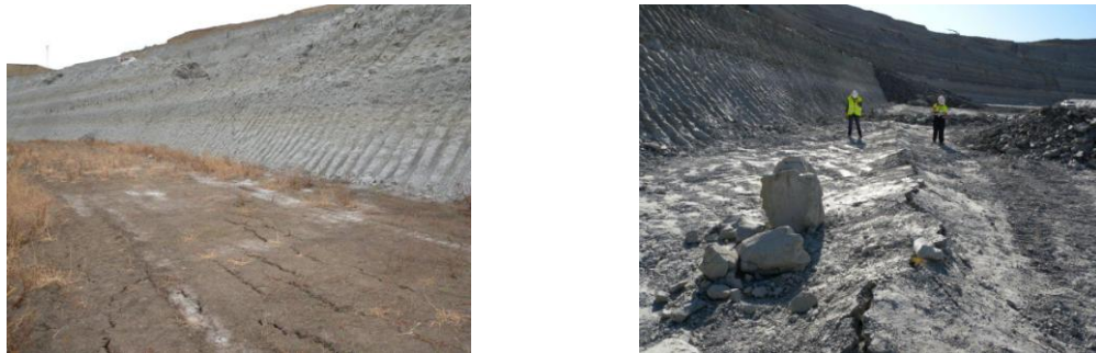
Figure 8. General views of the head and toe of the instability located at the North part of the pit.
