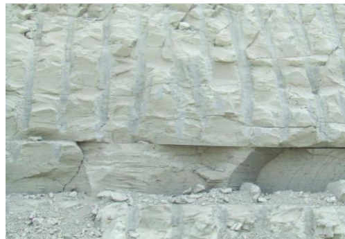
Figure 5. General aspect of the bedding in the marls and detail of one of those planes showing a millimetrical displacement.
