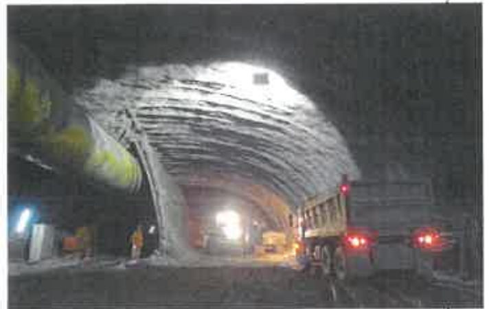
Above: The contractor used a hydraulic excavator, backhoe and wheel loader
