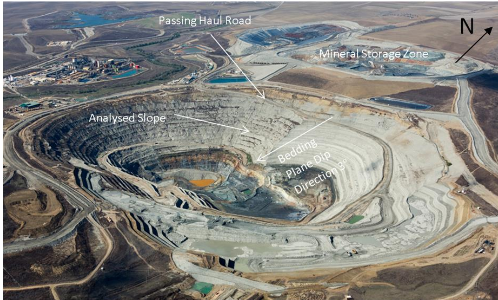
Photo 1. Pit layout showing slope in question.
