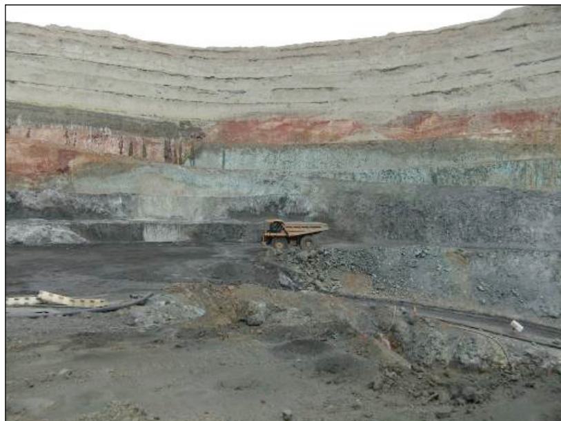
Figure 23 – Berm preservation via blast optimization in 2012
