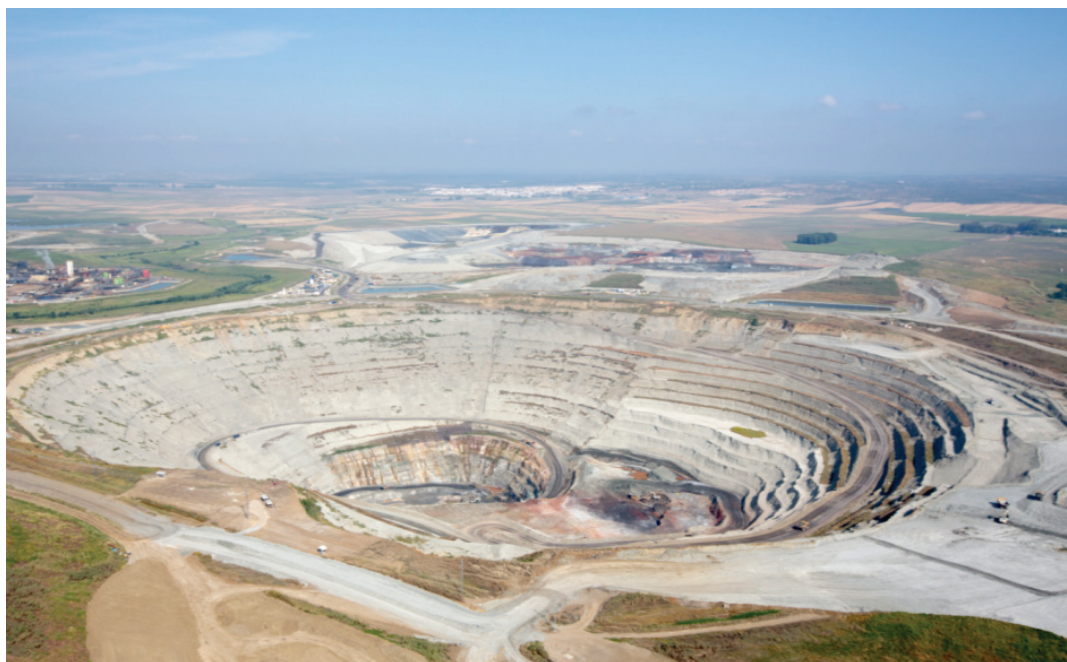
Figure 16 – Configuration of the pit in late 2012
