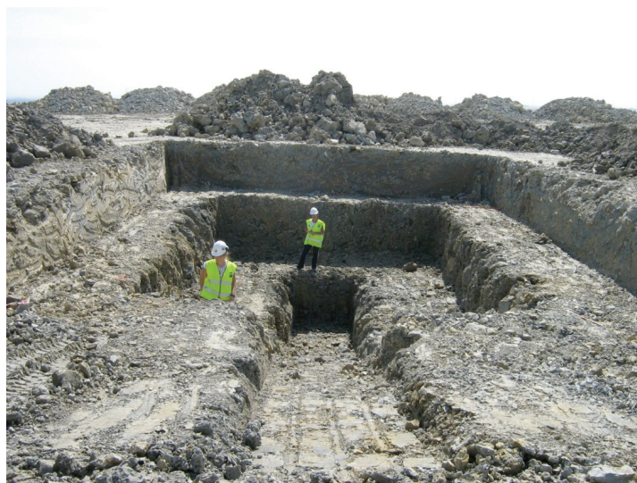
Figure 9 – Trial pit for the evaluation of the compaction value in actual dumps
