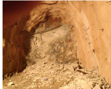
Figure 4: Rockburst at the face excavation in the headrace tunnel
