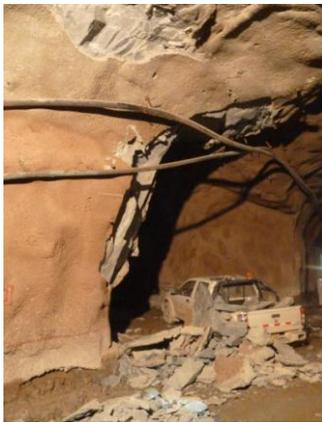
Figure 3: Rockburst in a drift near the Powerhouse Complex
