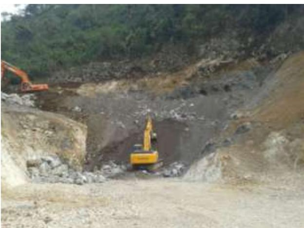
Photo 3. Tunnel 1, Adit portal in residual soils.
