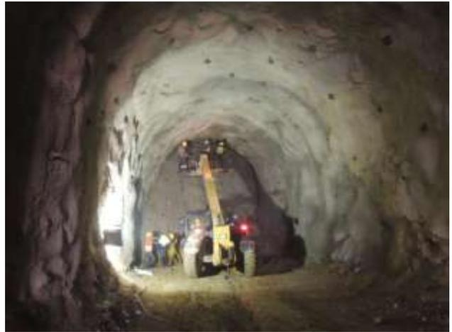
Photo 4. Charging the explosives at tunnel face T1.
