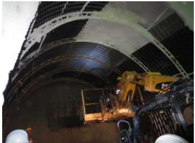
Photo 6. Installation of LG at a cave in T1.
