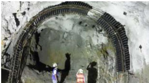
Photo 7. Treatment of a cave located at the roof in T1.
