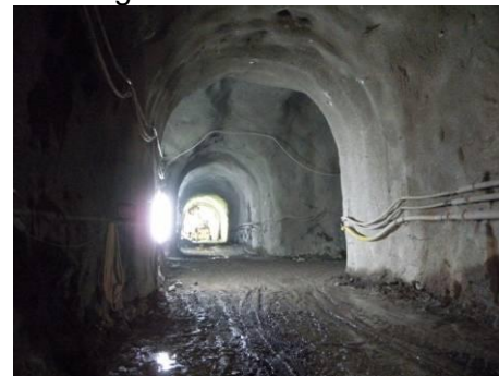
Photo 10. Junction T3-Tinguiririca Tunnel
