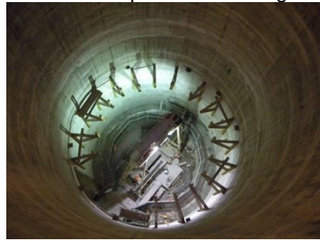
Photo 4. Surge Tank. Concrete Lining
