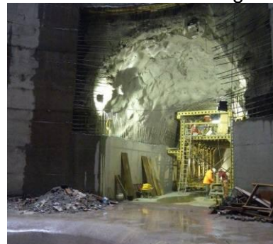
Photo 8. Junction of Tinguiririca Tunnel and Surge Tank/Pressure Shaft
