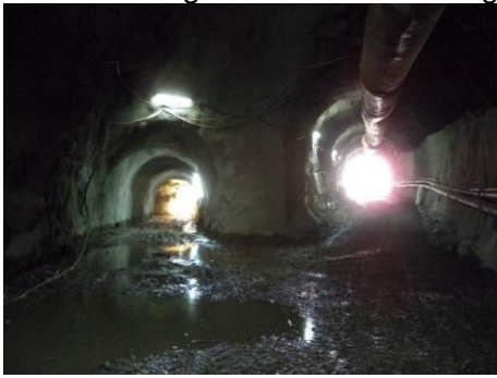
Photo 5. Junction H4-High Pressure Tunnel
