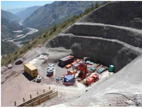
Photo 3. Surge Tank. Raise Boring
