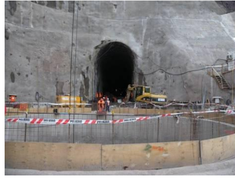
Photo 2. Portillo portal at the Surge Tank
