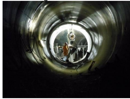
Photo 6. High Pressure Tunnel and Manifolds. Steel lining
