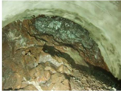
Photo 4. – Face at PK 1+48, showing the fault at the right hand side
