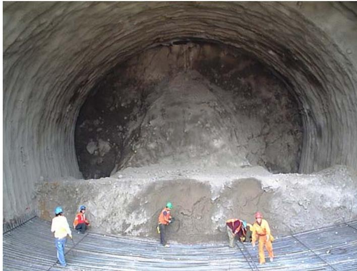
**Photo.3. – Detail of Tunnel C25. (South Portal) in colluvium soils.**
